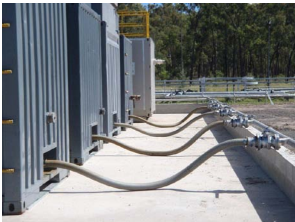
Process water facility constructed
