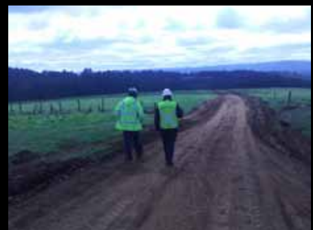
Establishment of access road, Mulpun, Chile
