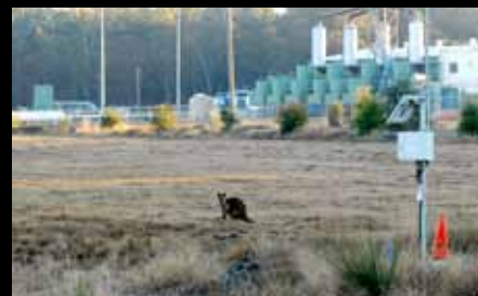
Power station at Bloodwood Creek
